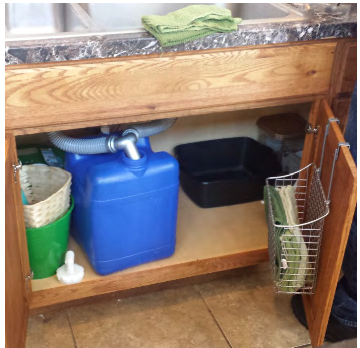
Figure 15. Temporary Infrastructure Accommodations
