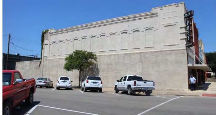
Figure 50. Northeast Corner of Knox St. and Dallas St.
