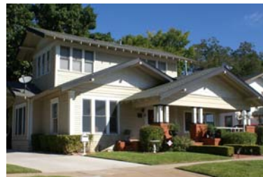
204 W. Belknap Street (Example of bungalow architecture)
